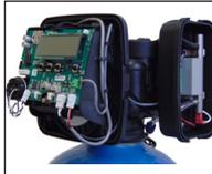
3. Route the grey control wire from the OzotechEOG into Clack® valve housing through the hole in the backplate, and through the strain relief channel above to keep wiring in place.
